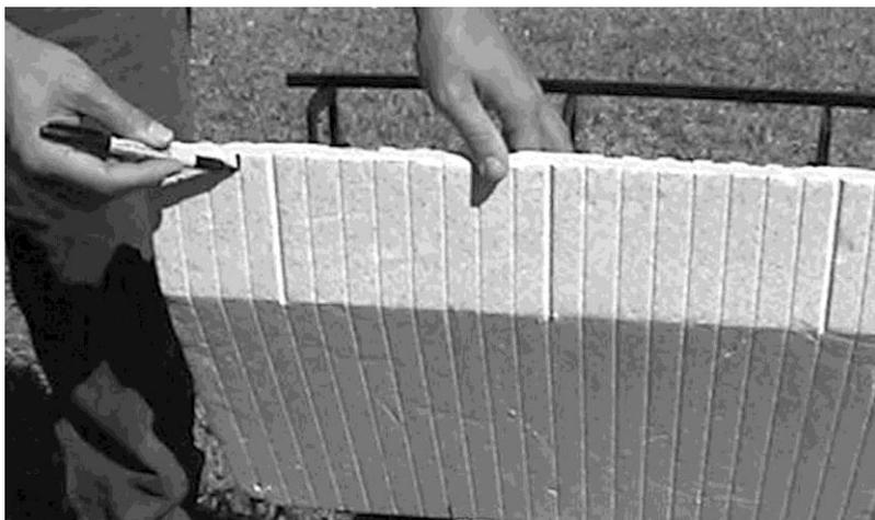
1. Place the CELBLOX<sup>®</sup> Brick Ledge panel over the corner block, lining up the third web of the brick ledge with the first web of the corner block.
