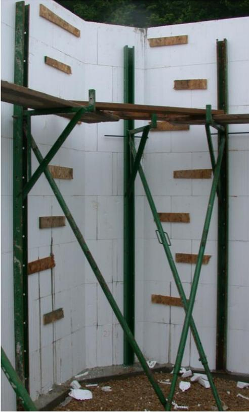
**NON-STANDARD JOINTS** are any vertical joints that are too close together or are not offset properly. Cuts wider than 4" should have strapping installed to span two webs in each direction and be installed on both sides. Scrap lumber, if long enough, or strips of OSB or plywood can be used for strapping these types of joints. The common seam, if used, should also be braced using this method.
