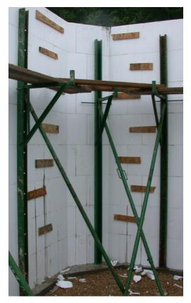
**NON-STANDARD JOINTS** are any vertical joints that are too close together or are not offset properly. Cuts wider than 4" should have strapping installed to span two webs in each direction and be installed on both sides. Scrap lumber, if long enough, or strips of OSB or plywood can be used for strapping these types of joints. The common seam, if used, should also be braced using this method.
